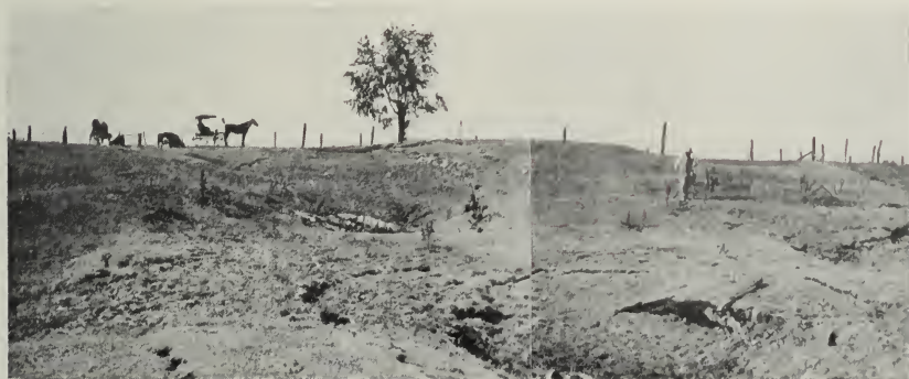
FIG. 21.—Side-hill breaks over shallow workings near Streator.
